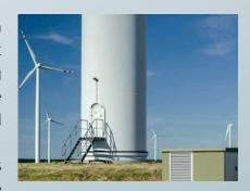
The heater bank was situated in a stainless steel enclosure external to the turbine
